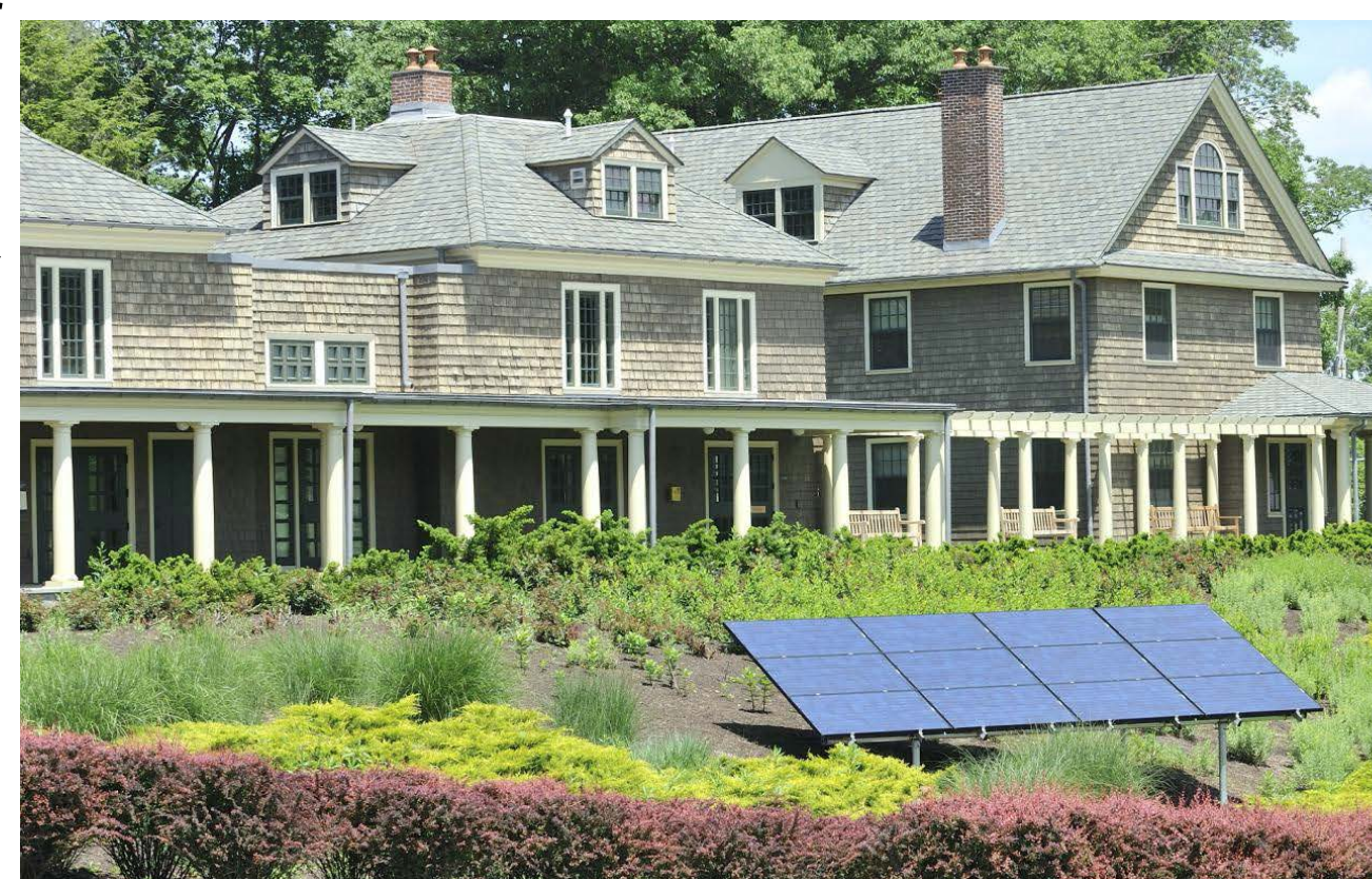
Fig. 1 Bryn Mawr's very own solar array located in front of Cambrian Row
